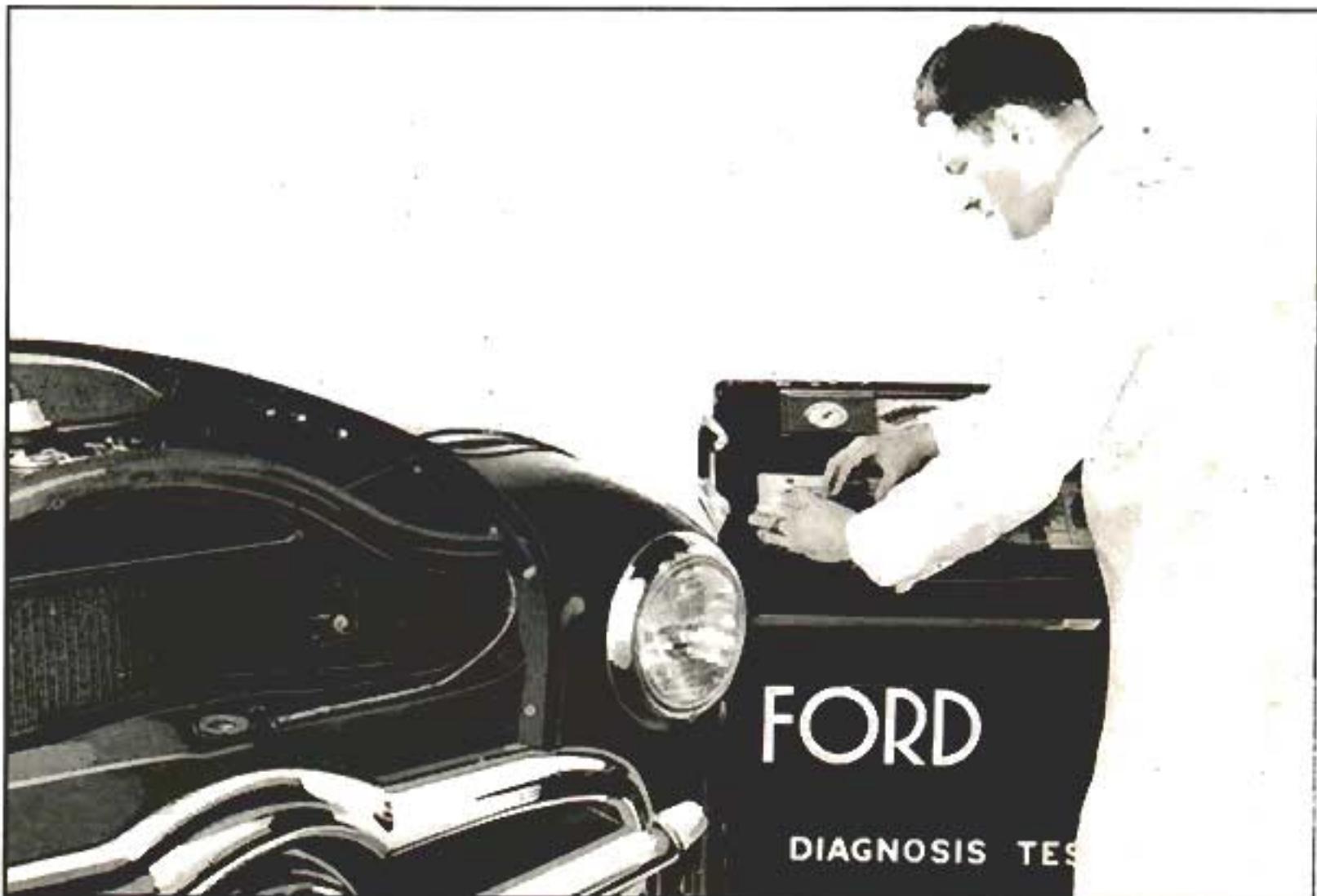
The Ford Diagnosis Test Set Aids in Engine Tune-up.
